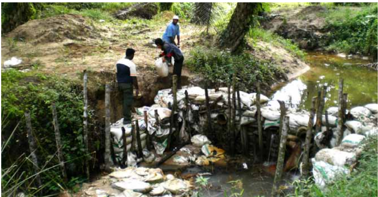
Water Conservation Dam
